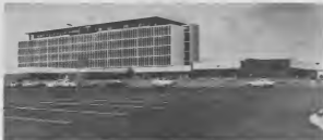
Accommodation : Airconditioned Building - 262 beds; Personnel - 350; Cost - over Fls. 28 Million; Parking : 450 cars; 10 Policlinics on East Side.
